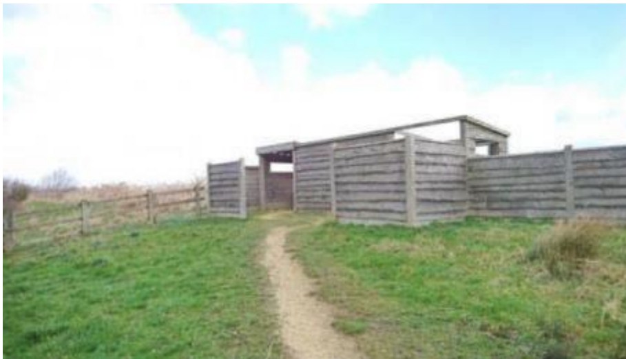
Ramp (no handrail) to the second viewing screen.
