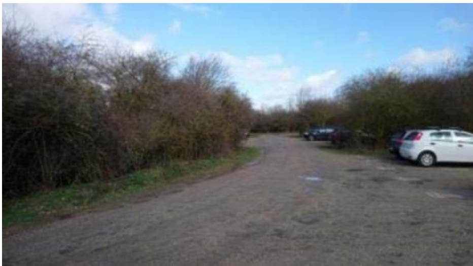
Car park, showing surface of compacted stone.
