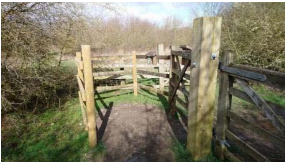
Kissing gate at main entrance with 130 cm clearance.
