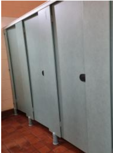
Doors to the cubicles in the toilets
