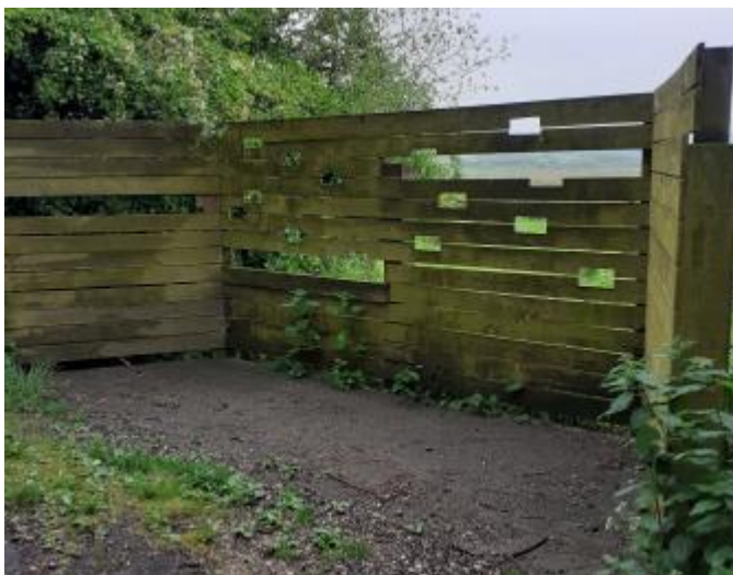
A viewing screen on the Arrow Lane Trail
