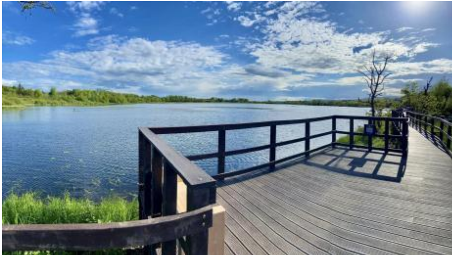
Boardwalk with viewing area/passing place
