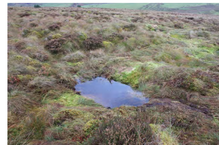
Completed peat dam at Muirkirk. Credit: Stephen Inglis
