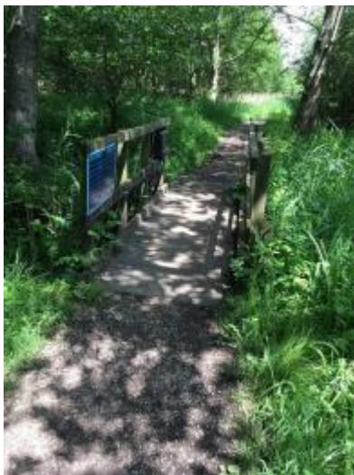
Lower trail footpath showing bridge
