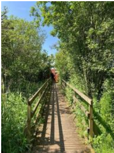
Access ramp to Eric Morecambe Hide
