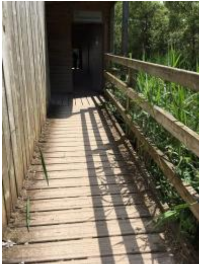
Causeway hide showing ramp and entrance to hide
