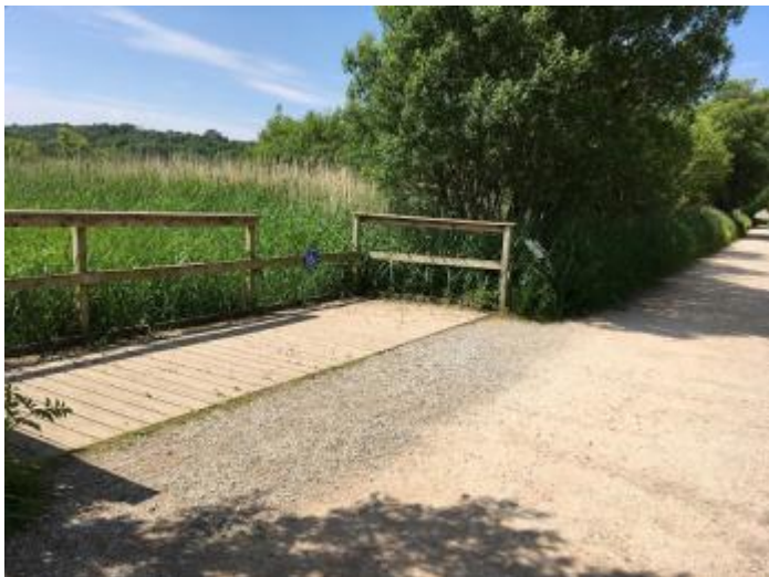
Lower trail bearded tit platform showing lowered viewing section for wheelchair users2
