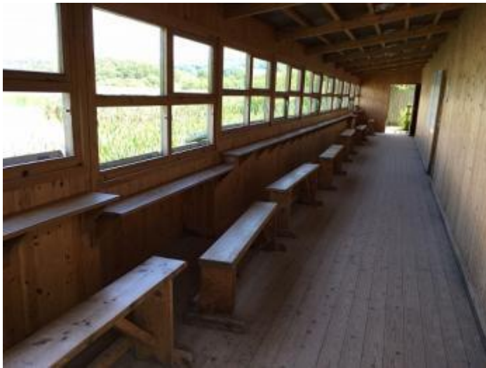
Causeway hide inside showing moveable benches and lowered viewing areas for wheelchair users
