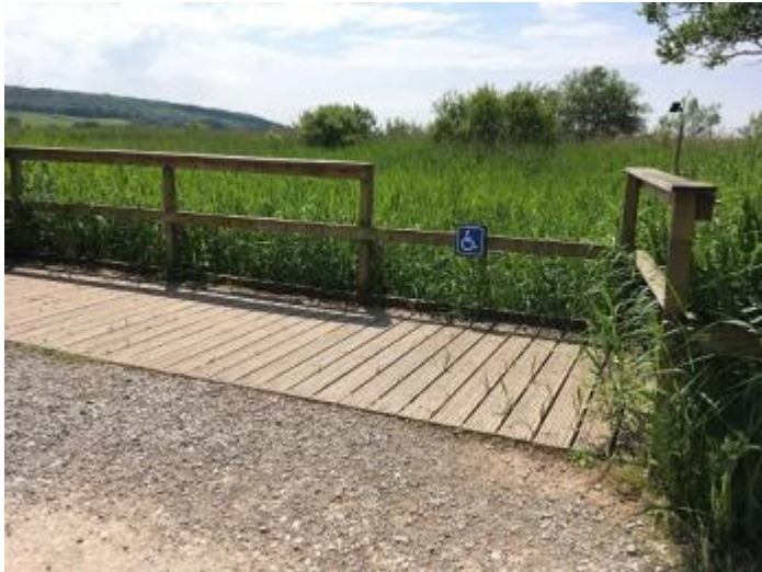
Lower trail bearded tit platform showing lowered viewing section for wheelchair users
