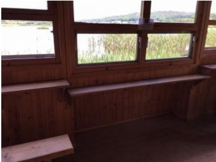
Causeway hide showing lowered viewing section for wheelchair users
