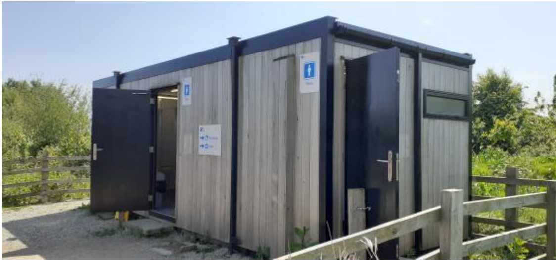
The toilet block at RSPB St Aidan's
