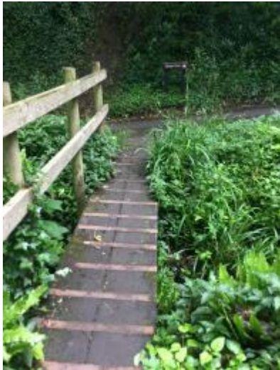
Bridge on Scarp Trail to road crossing.
