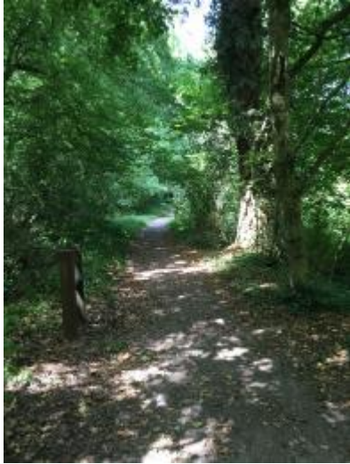
Compact dirt surface with loose surface path of Woodland Trail
