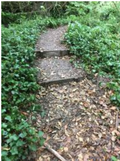
Steps on path to Scarp Trail from car park. Vegetation encroaching along path edges.
