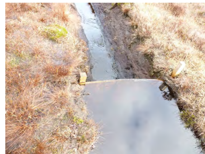
Wooden drain grip at Garron. Credit: Gareth Bareham
