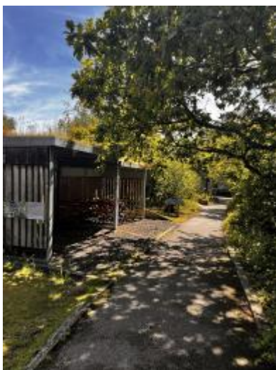
Ramped footpath from the carpark to the Visitor Centre
