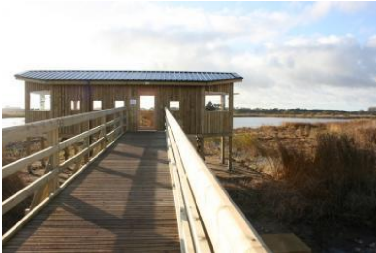
Approach to Island Mere hide showing the gentle slope of the ramp
