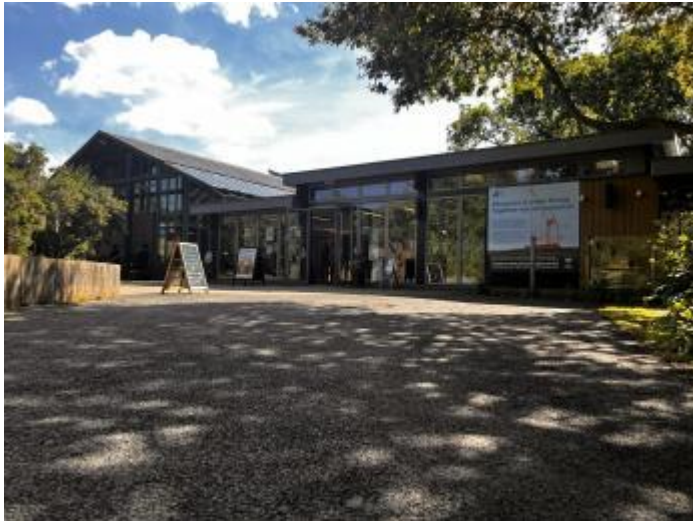
View of the Visitor Centre from the outside
