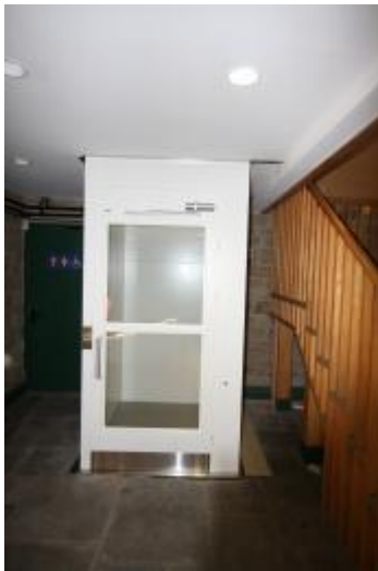
lift view from the visitor centre
