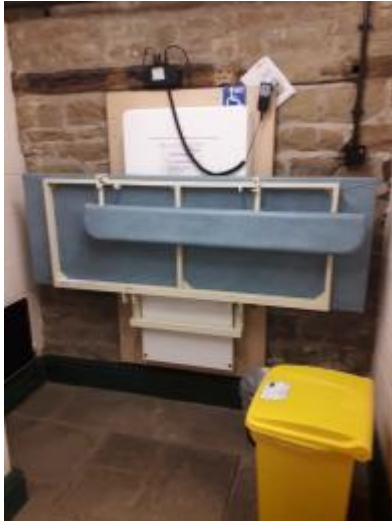
Changing table and hoist in the disabled toilet
