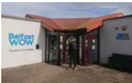
Solar panels at RSPB Belfast Window on Wildlife reduce our purchased electricity demands and lower running costs
