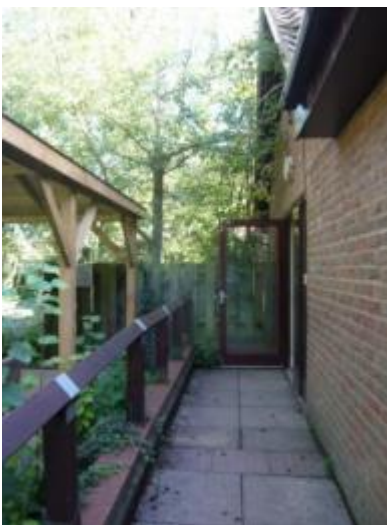
Rear Shop Access
